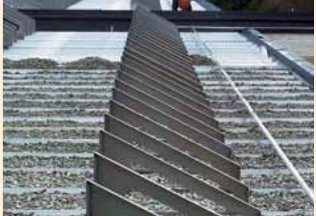
Linking the system with aluminium profiles, for example in a wind zone 2 location, with the adjunct "coast" and unfavourable structural conditions.
