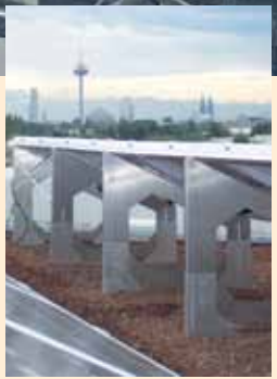
Linking the system with aluminium profiles, for example in a wind zone 2 location, with the adjunct "coast" and unfavourable structural conditions.
