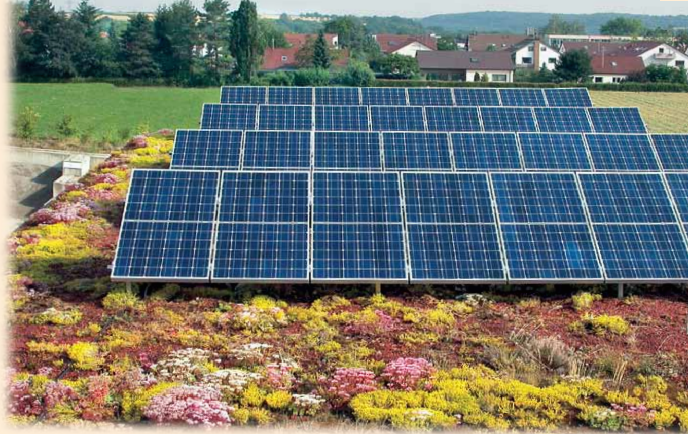
Roof of Pro Natur premises in Metzingen, Germany
