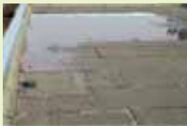
0°- roofs (ponding water)
