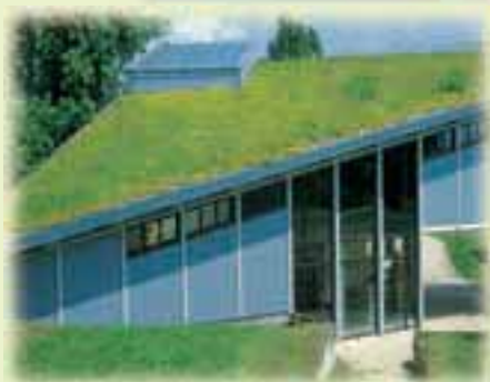
Green roofs often display remarkable designs. The photos demonstrate examples of pitched green roofs in Duisburg (above) or in Köngen at the Neckar river (left). Both green roofs were built with Floratec elements.
