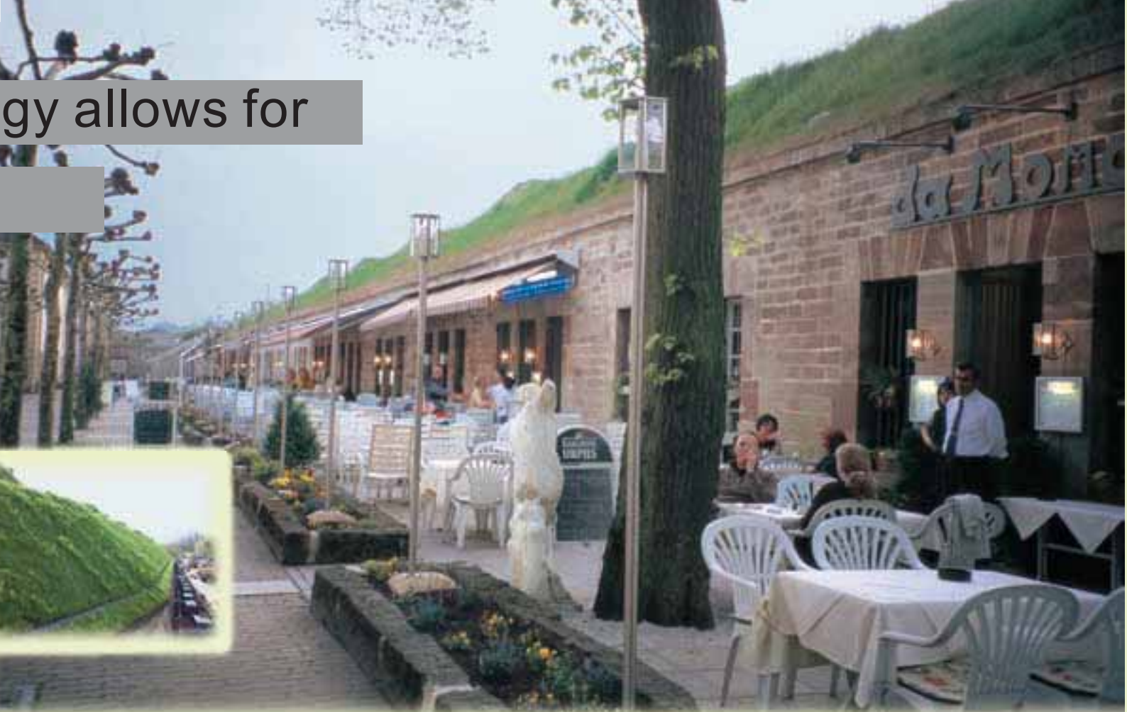
The “Prussian Casemats” in Saarlouis, at the beginning of the pedestrianized zone, hosts a number of restaurants.
