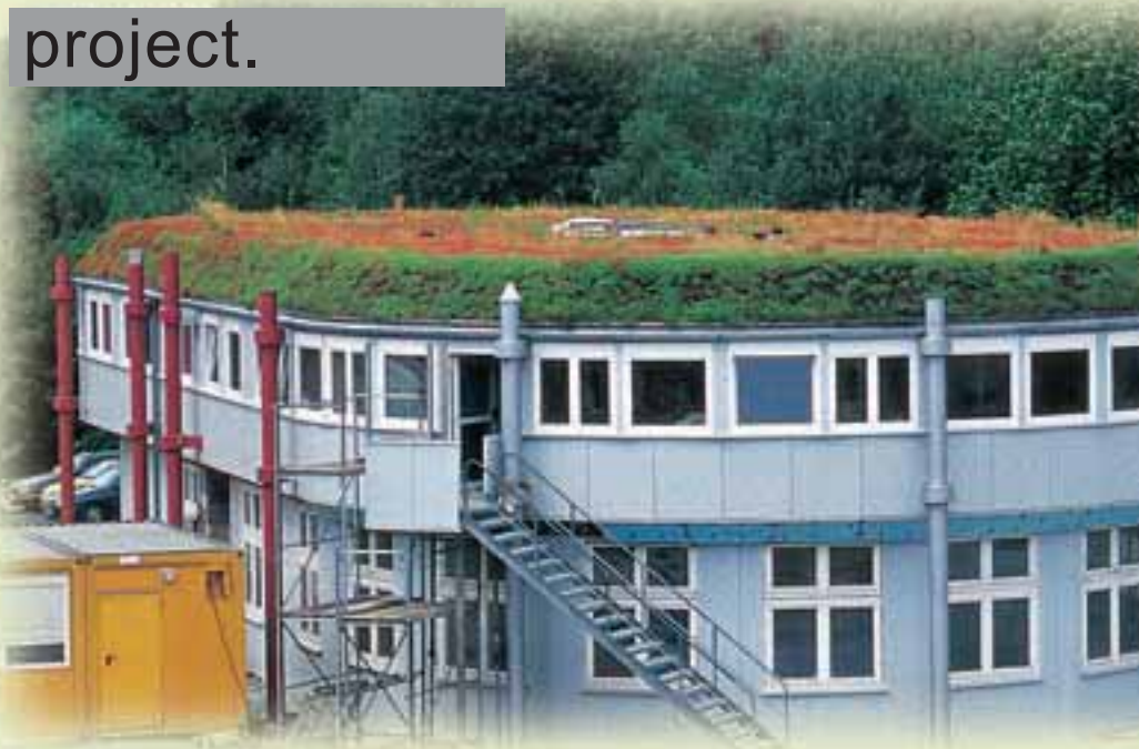
The basic construction of the new office building of the "Riedel-Baustoff-Recycling" in Moers, also called "UFO", is an
