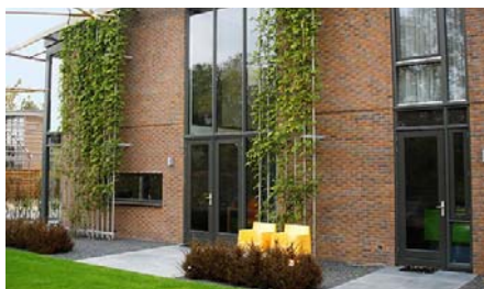
Left and right of the entrances, as well as above, are trellis for climbing plants available.
