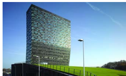
The green roof is rising steadily from the ground level during the office tower.
