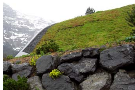
The sloped roof with newly-installed pre-cultivated vegetation mats.
