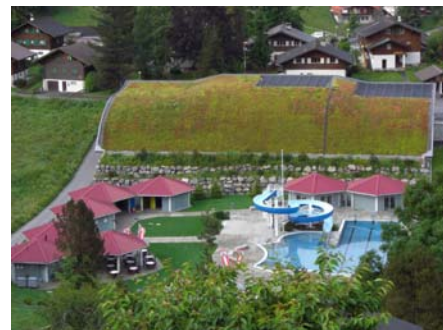
The collectors for warm water can be seen at the top right of the extensive green roof.
