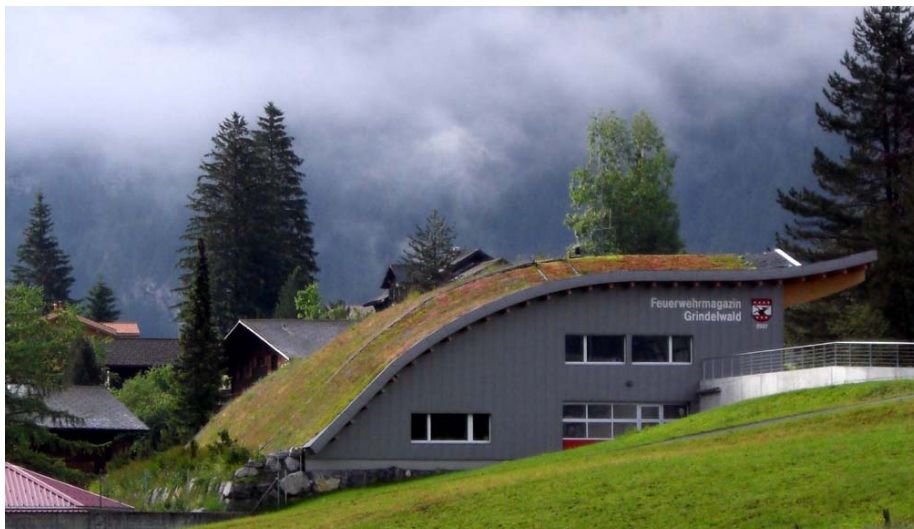
The Grindelwald fire station is at one with the surrounding mountainside.
